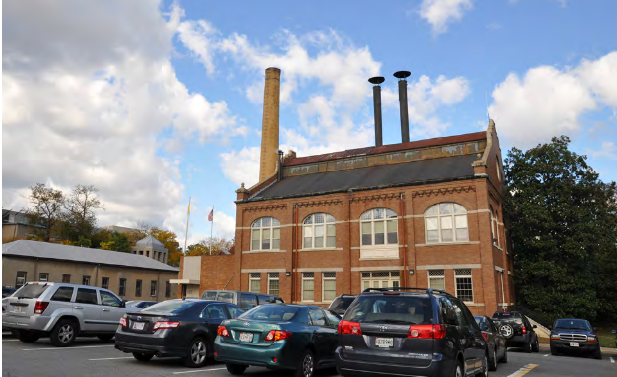
Existing Power Plant
